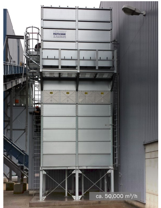
MultiStar stirrer device filter • biomass power plant
