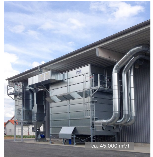
MultiStar jet filter • prefabricated house production
