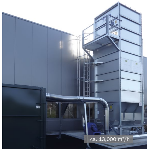
MultiStar valve filter with container feeding
