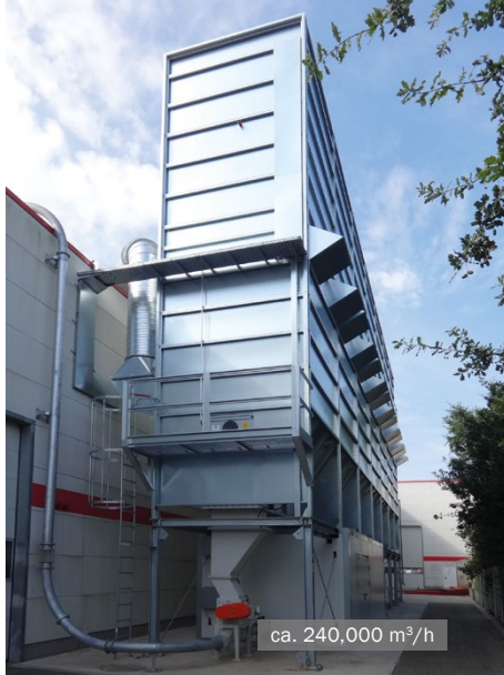
MultiStar reverse air flow filter • kitchen manufacturing
