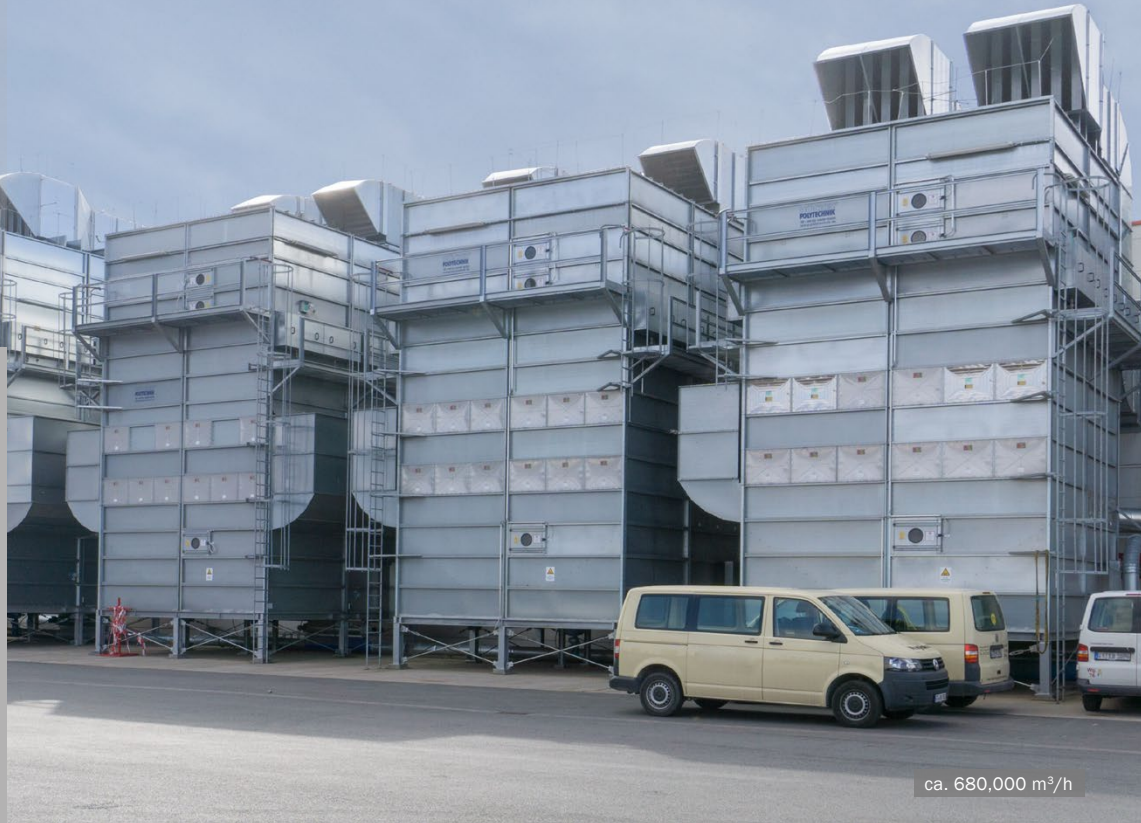
MultiStar stirrer device filter with jet cleaning • kitchen manufacturing
