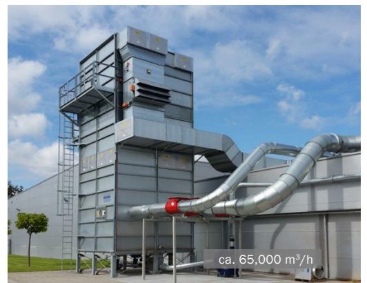
MultiStar stirrer device filter • plywood production
